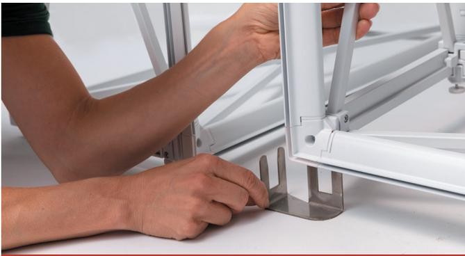
2. Lift one frame and slide the connector in the slot of the outer hinge.
